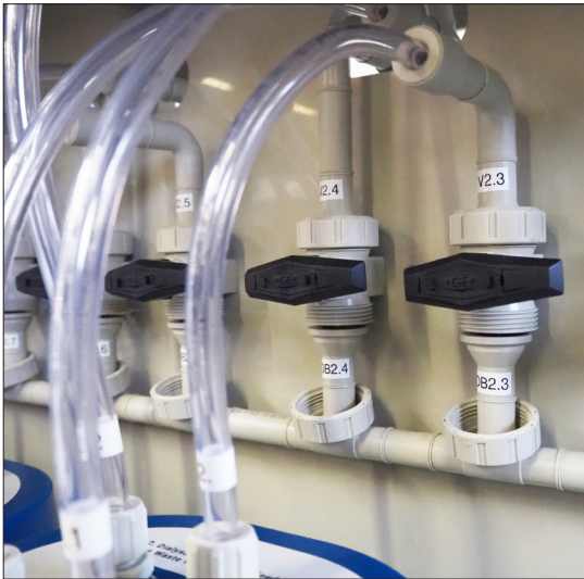
Figure 11: Loosening screw caps
