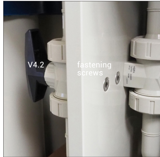
Figure 12: Mounting drain valves
