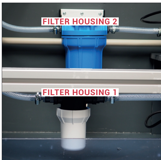
Figure 10: Filter housing in the system
