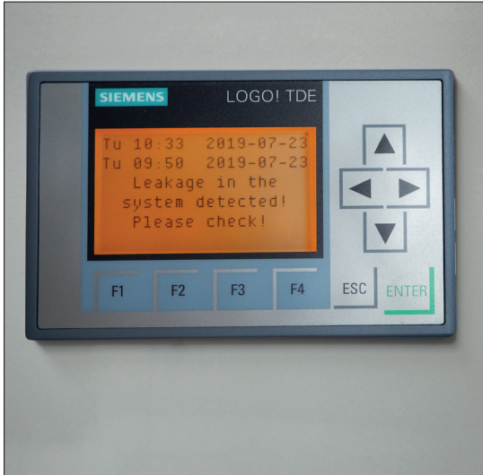
Figure 20: Example of a fault message
